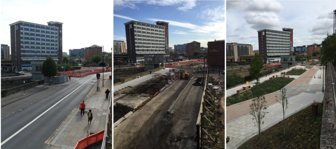
Figure 6 - Grey to Green example before, during construction and after (source: https://www.greytogreen.org.uk/background )
